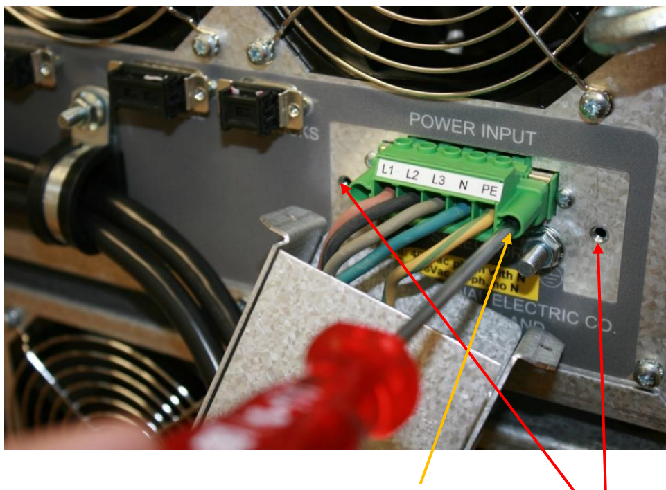
Figure 9: Tightening the input mating connector to BPS. Metallic cover's fastening
